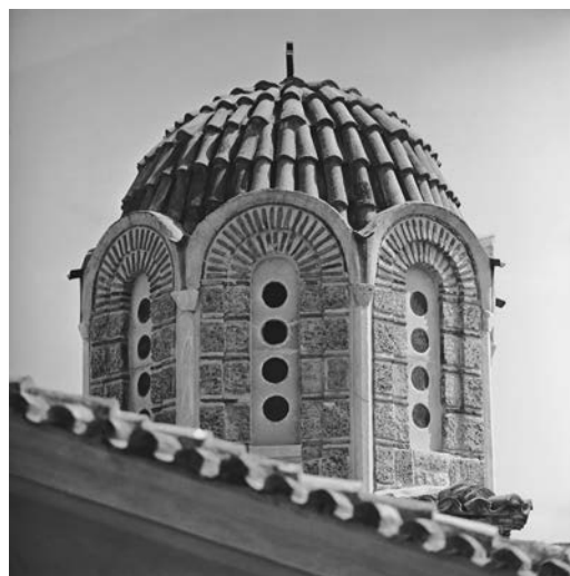
Figure 197 Hagios Nikolaos Rangavas. Dome after restoration.
